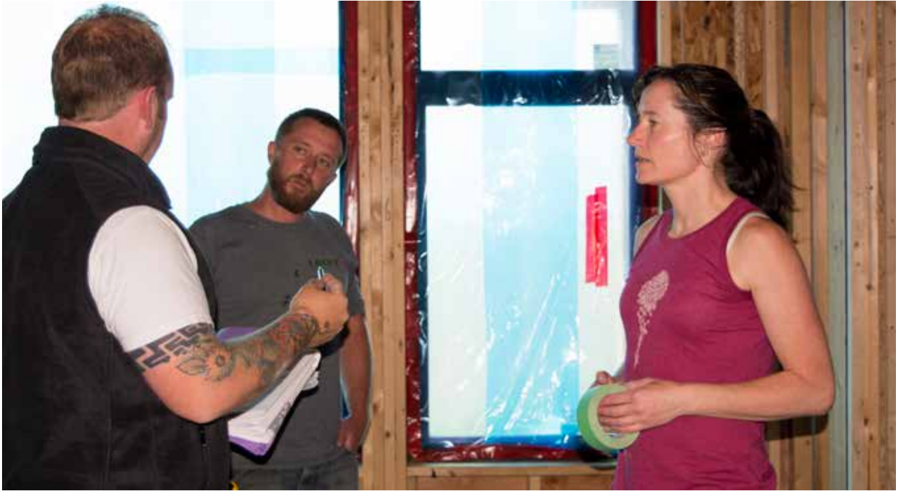
FVRD Building Inspector, Greg Price, reviewing his inspection report with Lacey Developments Construction Manager, Claire Seymour and Project Manager, Landon Hood.
